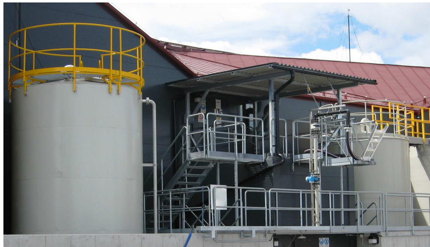
One out of seven stainless process vessels for the manufacture of special products at a paper mill in northern Sweden. Height ca 10 meter, diameter ca 2.5 meter, the conical part is ground and electropolished on the inside. Material: 1.4404/316L.
